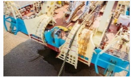
INTER-ARRAY CABLE EXCHANGE
